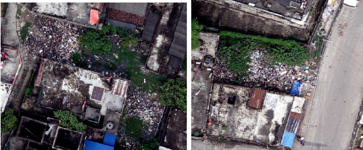
Fig: haphazard solid waste disposal in Janakpur
